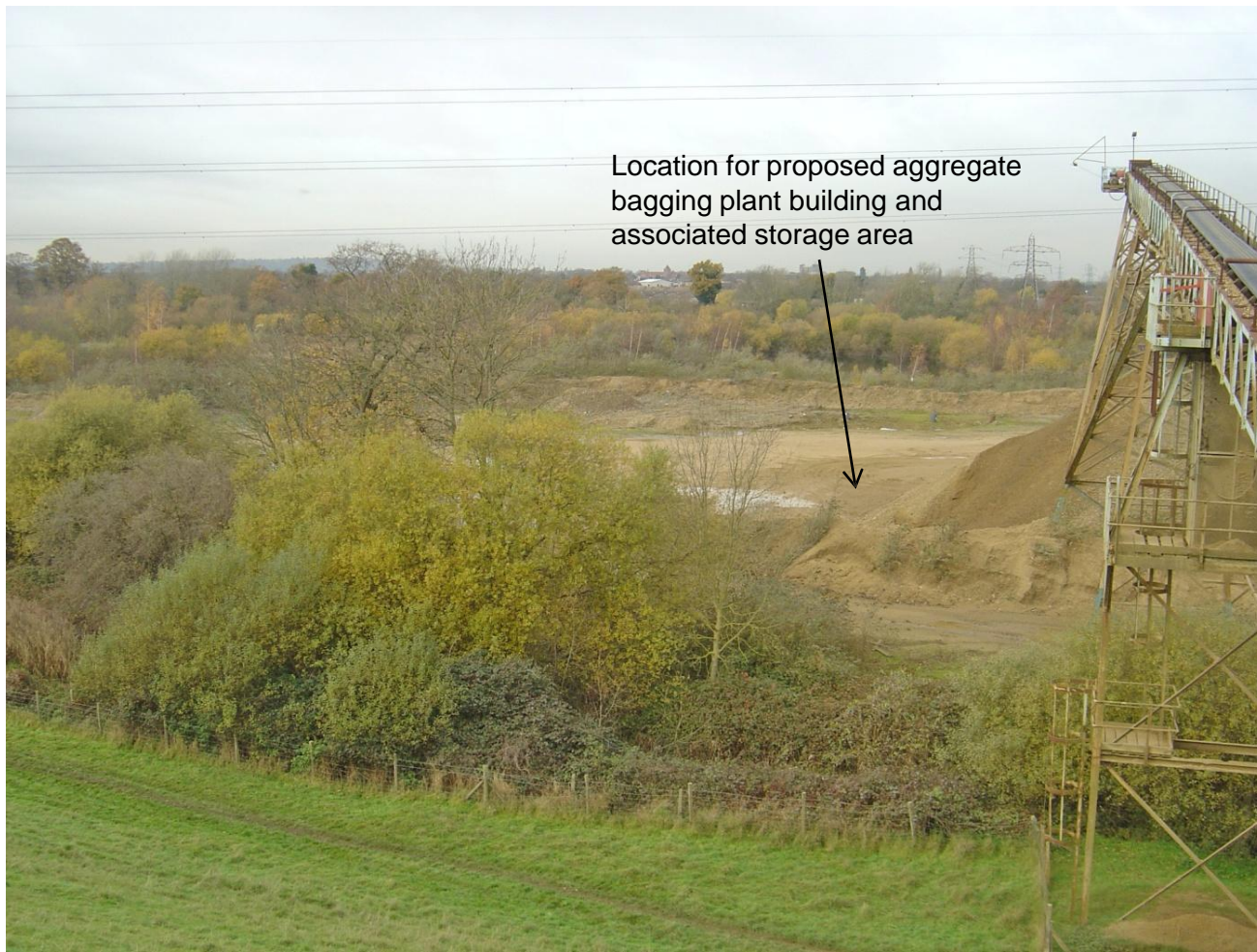
Figure 11 : View over southern part of existing Queen Mary Quarry processing plant site taken from reservoir embankment (location for proposed aggregate bagging plant).
