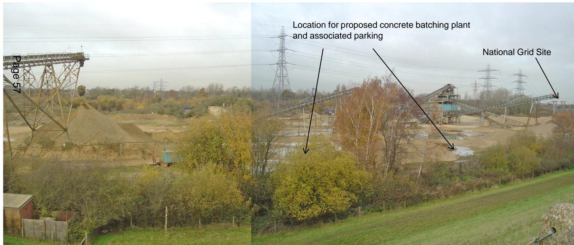
Figure 10 : View over existing Queen Mary Quarry processing plant site taken from reservoir embankment (location for proposed concrete batching plant and mixer truck parking area).
